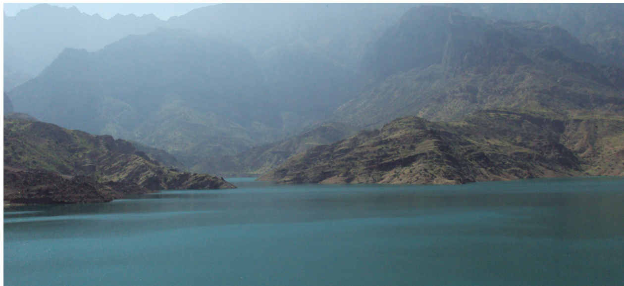
Wadi Diqah Dam reservoir, Oman, 2011. Source: Ihab Jnad.
