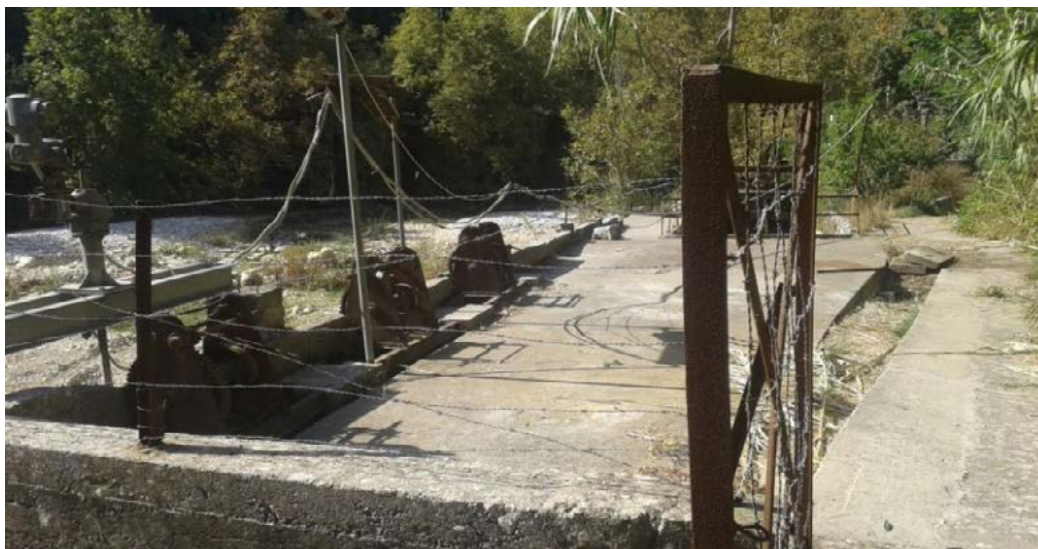
Jeita Dbayeh Conveyer, photo by Tom Zoghby.
